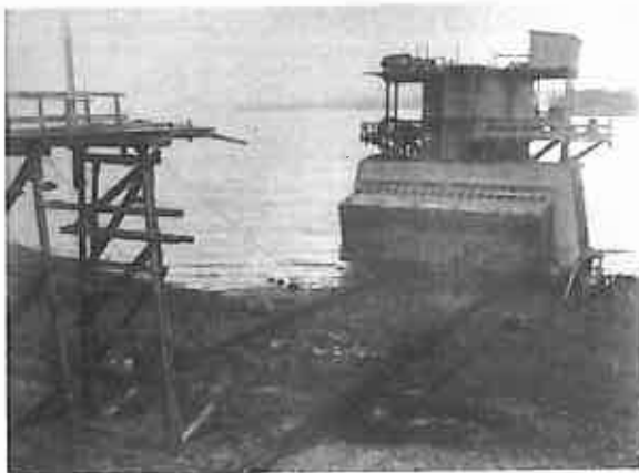
fig. 11 – 19.08.1926. 19.08.1926. Launching of Lancement du caisson.
