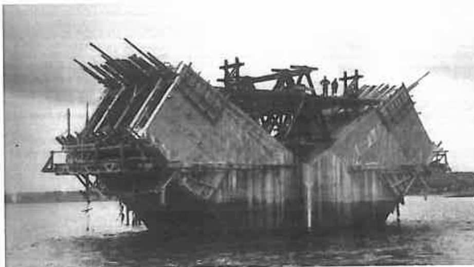
fig. 13 – 2.09.1927. 2.09.1927. Construction of Construction des amorces arch bases on a pier.
