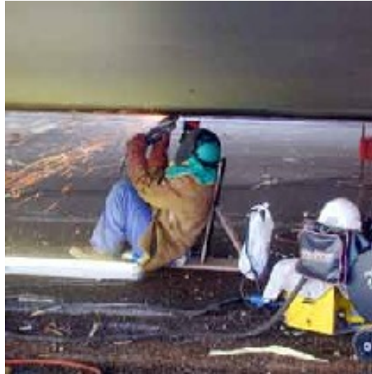
Welding the first deck member (photo ASCO-TP)
