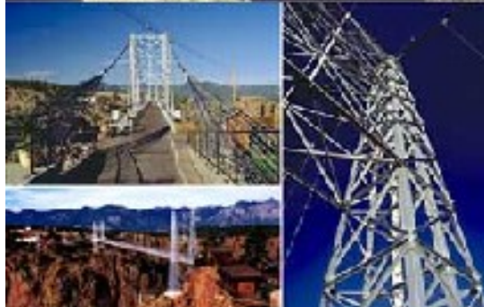
The Gorge Bridge in Colorado
