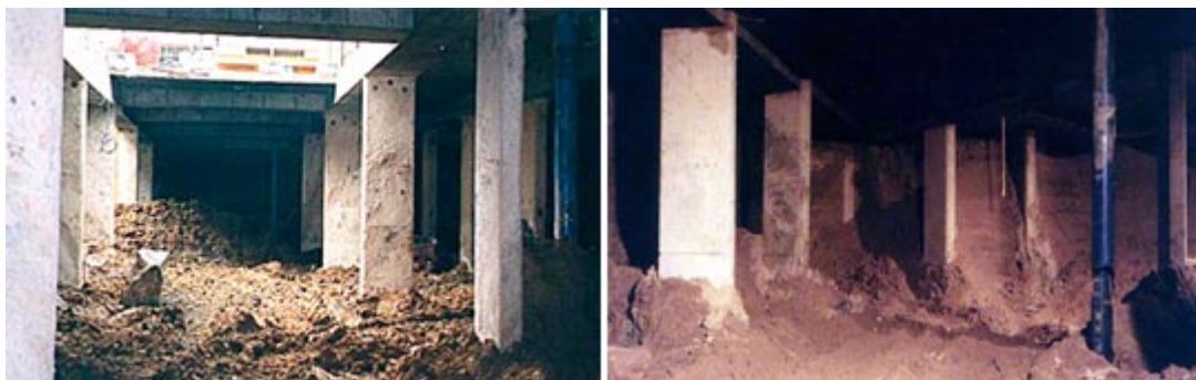
Construction parking Levallois
